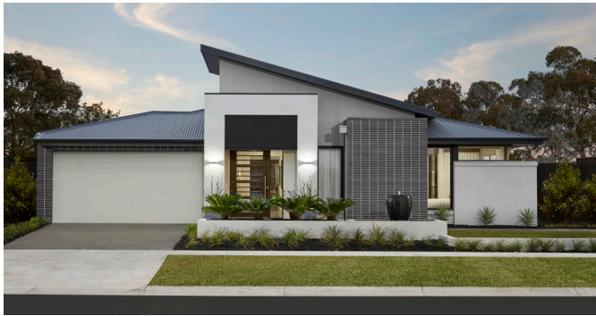
Skillion Roof - Metricon Homes (Botanica)
