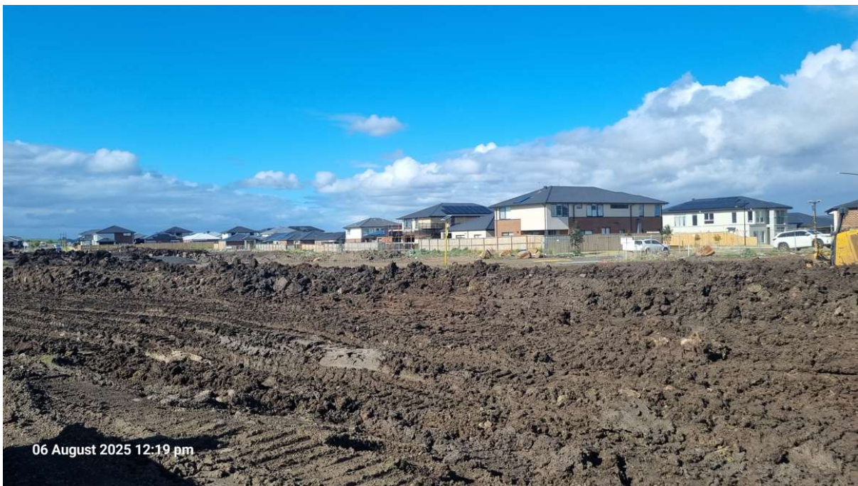
Figure 4. Site Photo – Olivine Estate Stage 26
