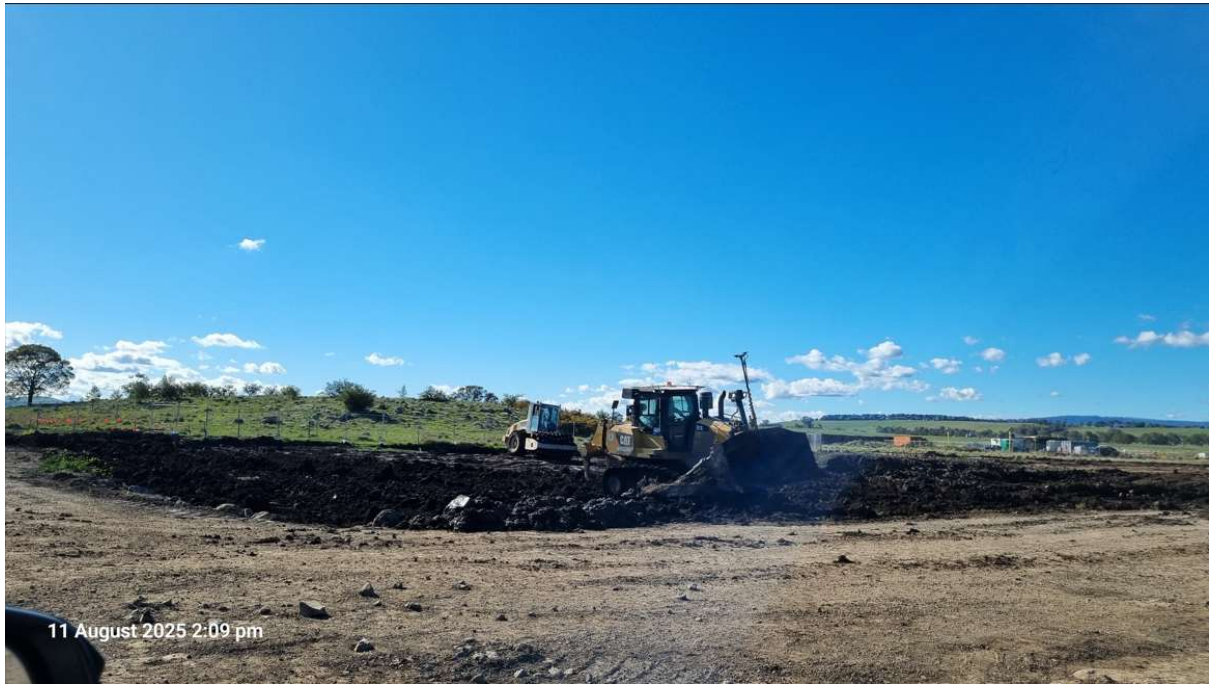
Figure 7. Site Photo – Olivine Estate Stage 26
