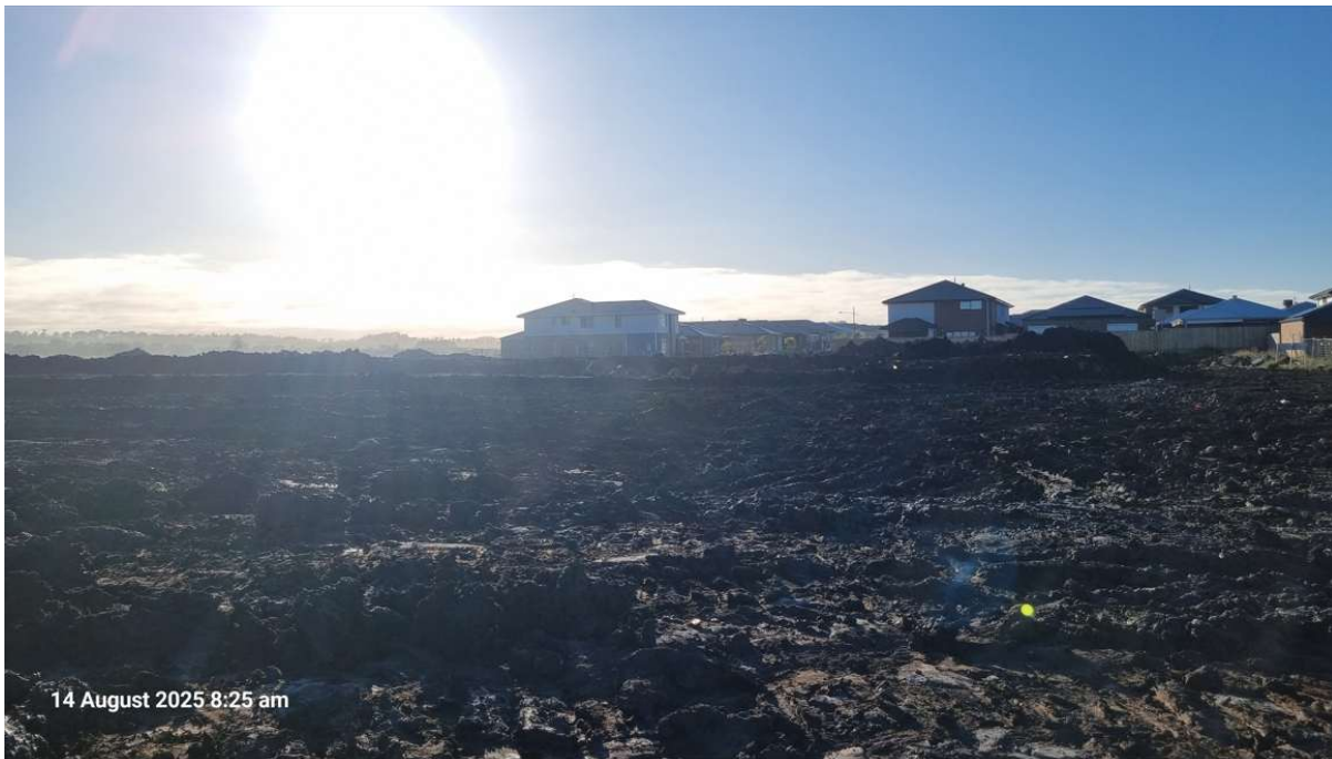
Figure 10. Site Photo – Olivine Estate Stage 26
