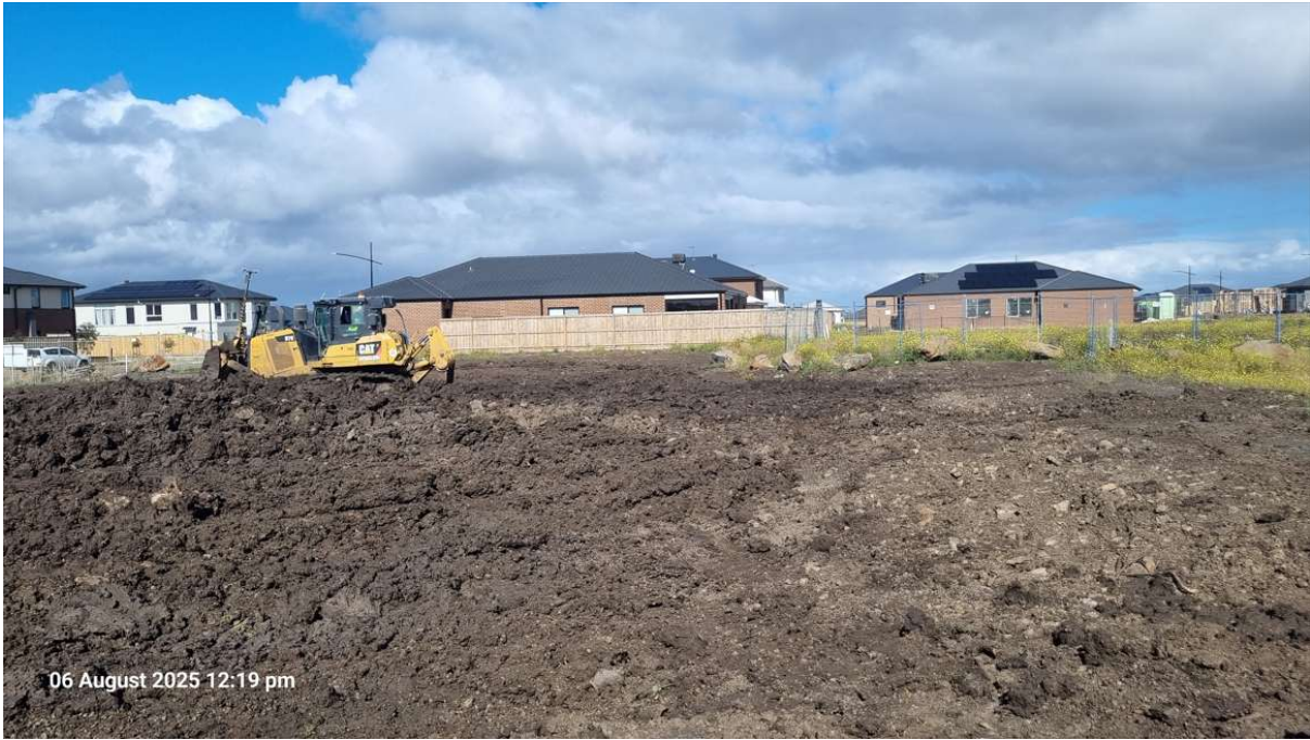
Figure 3. Site Photo – Olivine Estate Stage 26
