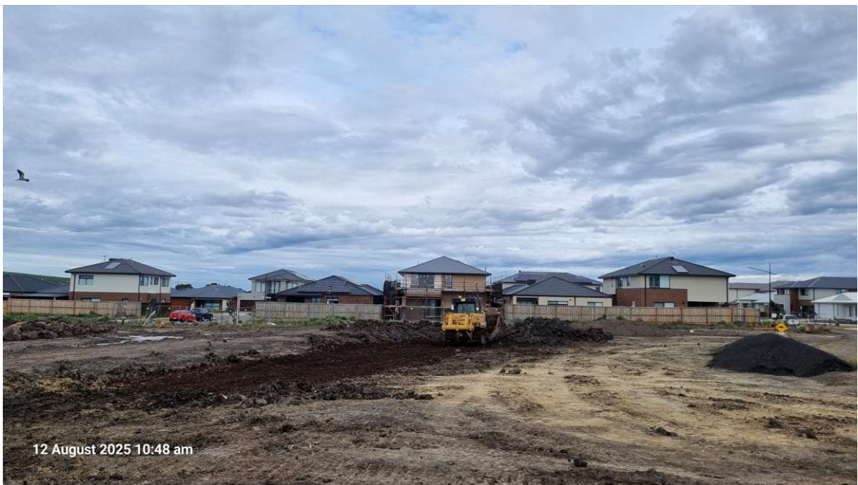
Figure 8. Site Photo – Olivine Estate Stage 26
