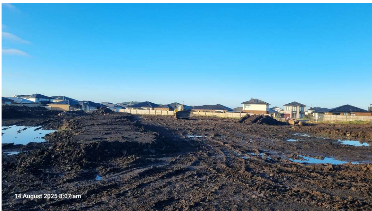
Figure 9. Site Photo – Olivine Estate Stage 26
