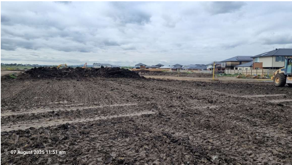
Figure 6. Site Photo – Olivine Estate Stage 26
