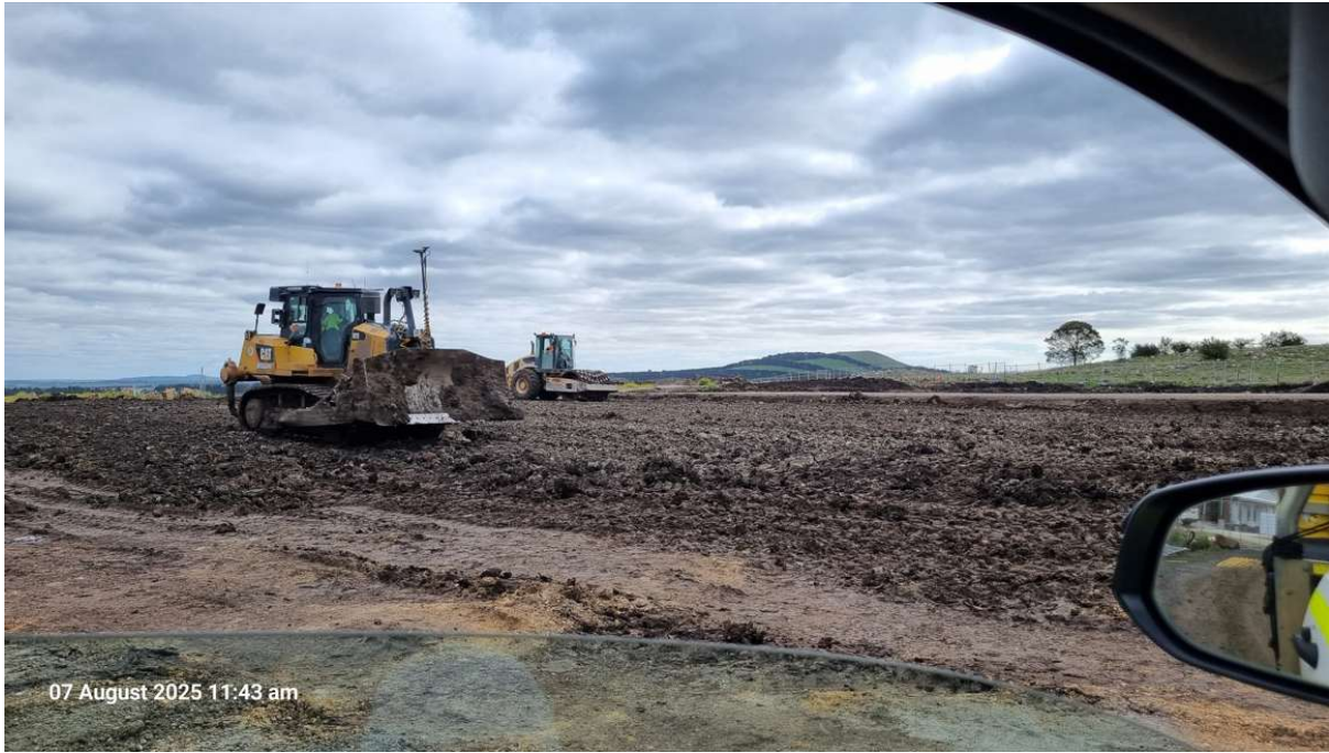
Figure 5. Site Photo – Olivine Estate Stage 26
