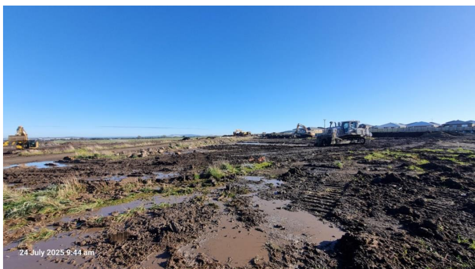
Figure 1. In-Situ Clay Structural Fill
