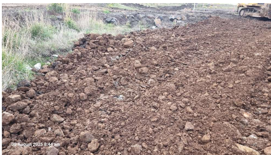
Figure 2. Oversize Aggregates on stockpile
