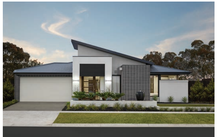
Skillion Roof - Metricon Homes (Botanica)
